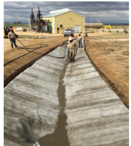
Armor protection using Concrete Cloth GCCM for a drainage ditch.
